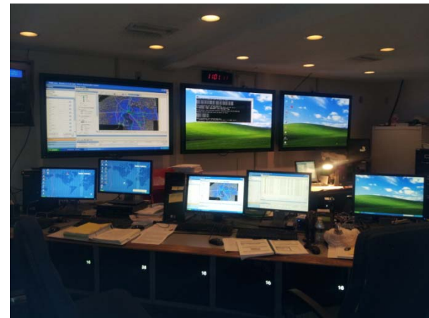
City of Jacksonville Signals Office
