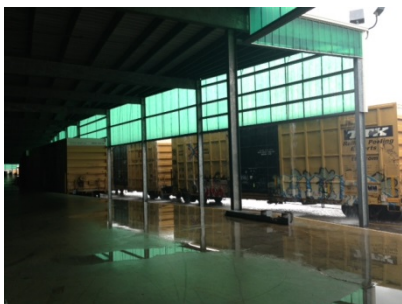
Above, pictures from the Seaonus warehouse at Jaxport's Talleyrand facility
