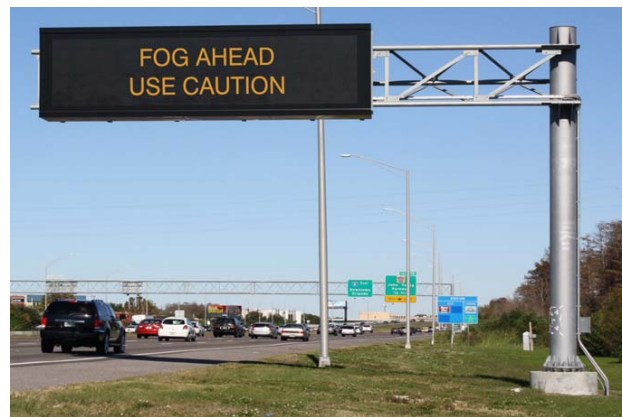
Above: New DMS signs on I-75 to notify motorists of adverse conditions and incident; below: Infrared cameras to monitor low visibility conditions. Photos courtesy of FDOT.
