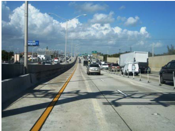
Above: FDOT District 6 (Miami) Express Lanes
